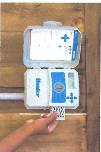
Smart Controller w/ rain/freeze sensor
